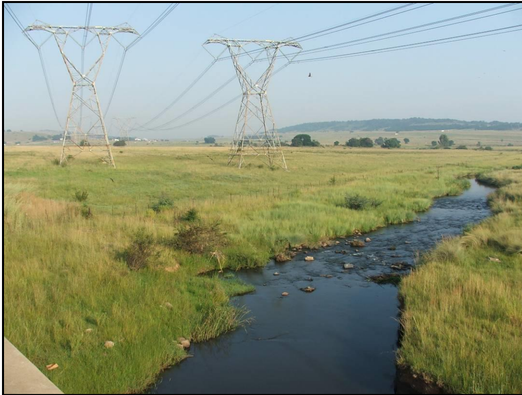
FIGURE 57: VIEW OF THE EXISTING POWER LINE ON SITE
