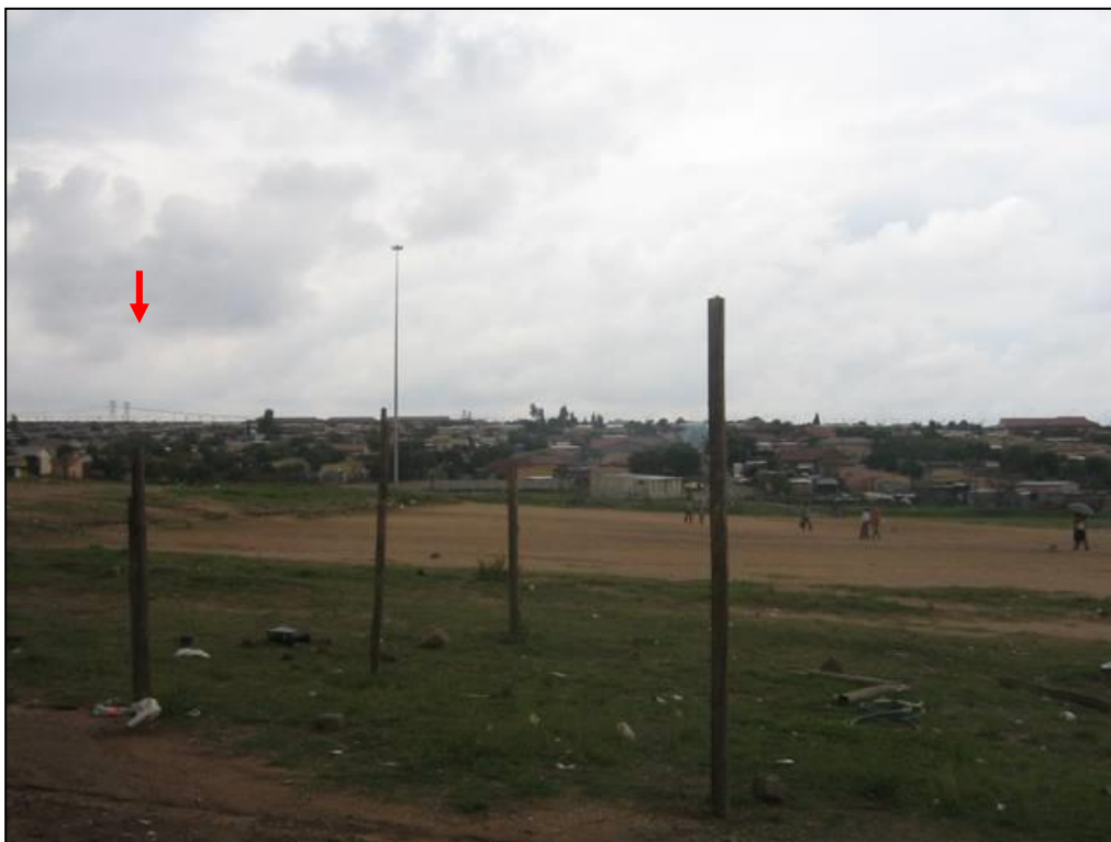
FIGURE 71: OLIEVENHOUTBOSCH WITH CORRIDOR IN DISTANCE (PARALLEL TO EXISTING TRANSMISSION POWER LINES)
