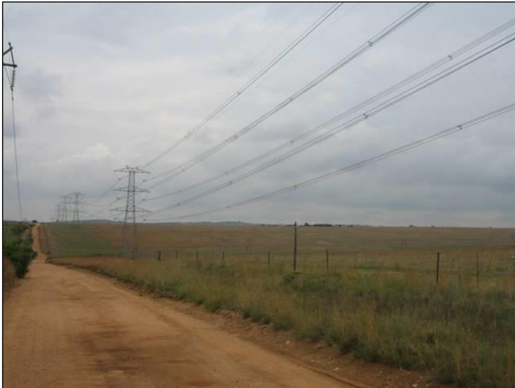
FIGURE 70: LAND USE SURROUNDING PROPOSED ROUTE CORRIDOR NORTH OF THE N14
